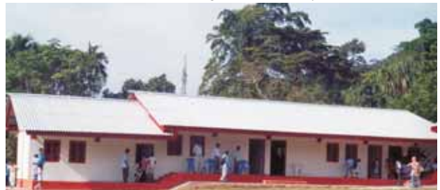
Reconstructed school at Korang Nalah A & N by BJS
