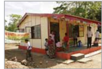
Re-constructed Public Health Service Centre (PHSC) by BJS at Harmindar Bay, Hut bay, A & N-2005
