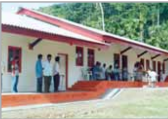
Newly reconstructed school by BJS at Korangnallah, Middle Andaman-2005
